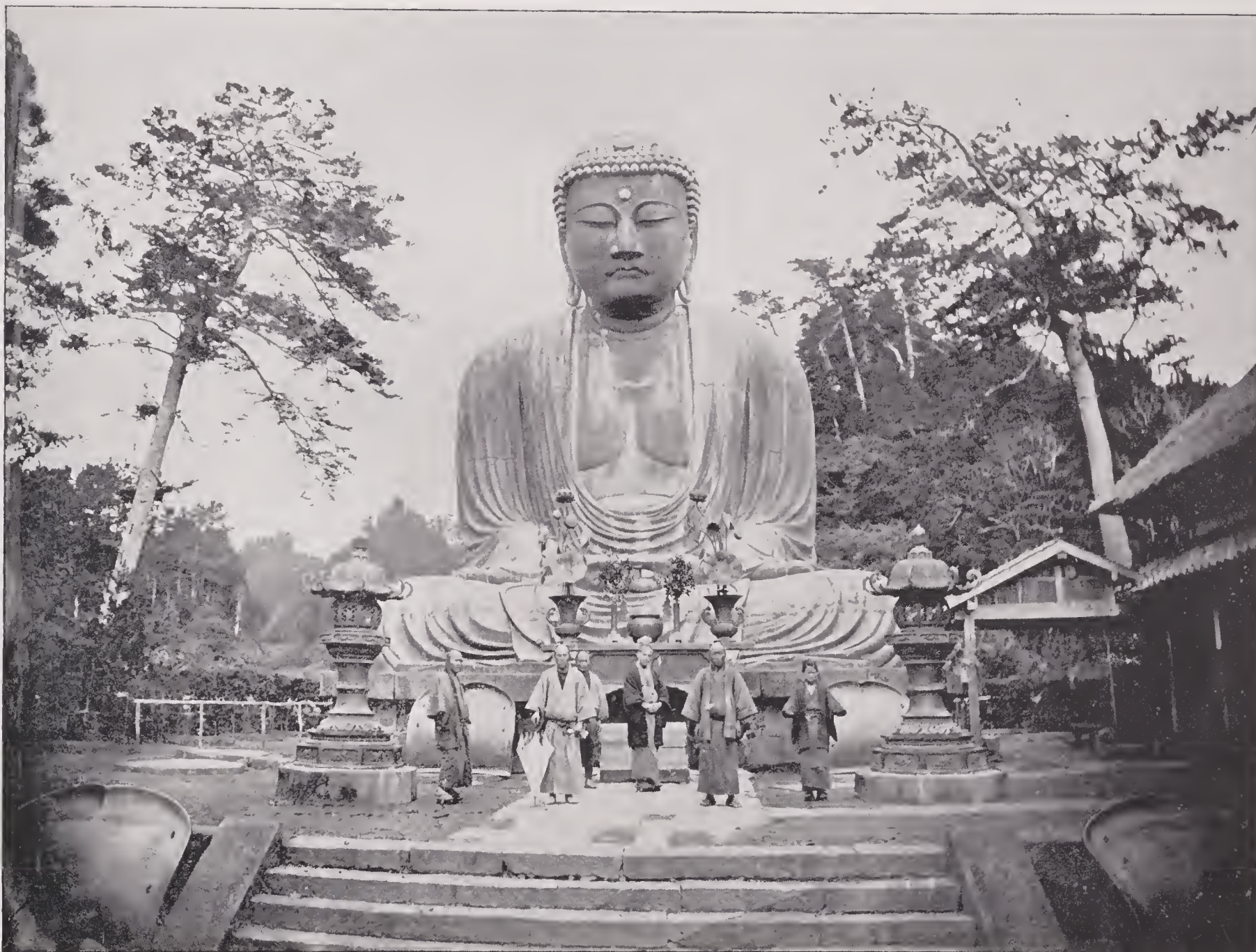
GREAT BUDDHA, KAMAKURA, JAPAN.—This colossal figure, of great antiquity, is in a sitting posture and is forty-seven feet high. It was cast on the spot, in sections of about six feet in height, forming one huge mass of metal, in which the divisions of the several castings are distinctly visible. The figure represents Buddha in meditation and is full of dignified repose. A large jewel is placed in the middle of the forehead, from which light is supposed to beam, and is significant of Buddha being "The Light of the World." This wonderful piece of work was, after eight failures, accomplished in 749 by Takusho, an artist from Corea, and is marvelously perfect and well preserved.
